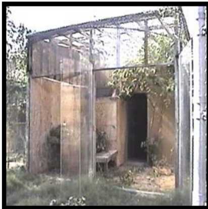
Clear hard plastic covering (viewed from yard)
